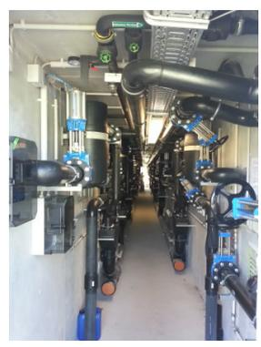
Figure 1: The distribution system for loading and O&M of the DWWT-technologies at the BDZ.
