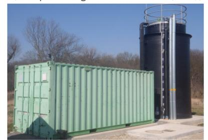
Figure 2: A dosing station (22 m<sup>3</sup>) and a container with a mixing tank inside.
